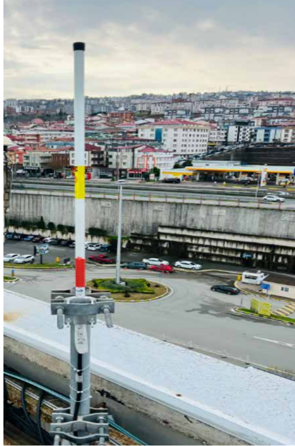
ADS-B antenna installed at Trabzon Airport
